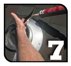
Step 7: Caulk the Shingles to the Flashing
