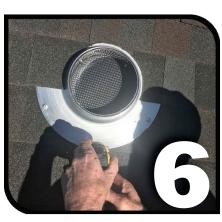
Step 6: Attach Flashing
