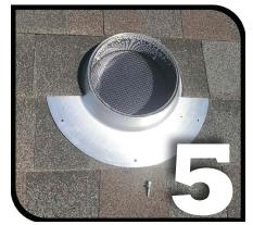
Step 5: Caulk and Insert **Flashing**
