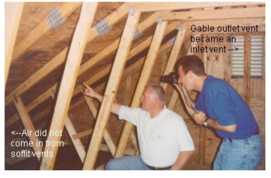
flowing, along the entire underside of the roof's sheathing, gathering up and removing water vapor.
