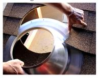
Using the **hex bit** on the **electric drill**, fasten the **flashing** to the roof with **#10 x 1 ½**" **flashing screws**. Screw the exposed predrilled holes first and fasten rest of screws about 7" apart.
