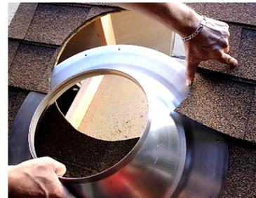
Using the hex bit on the electric drill, fasten the flashing to the roof with #10 x 1 1/2" flashing screws. Screw the exposed predrilled holes first and fasten rest of screws about 7" apart.
