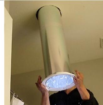
Slowly fasten **ceiling ring screw tabs**. **Ceiling ring** has self-tightening wing nuts to connect with drywall. **Do not overtighten**.
