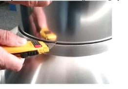
Install **dome assembly** over **flashing** lip and fasten with **#8 x** <sup>1</sup>/<sub>4</sub>" **dome screws**.
