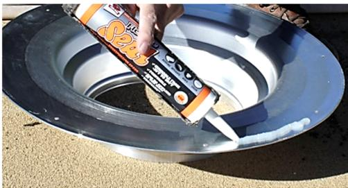
Slide flashing at cut slits (slightly lift to avoid smearing sealant) under the shingles and tar paper, center the flashing over the roof hole.
