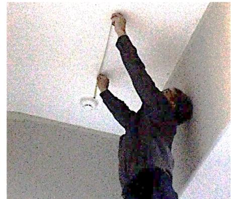
Use a **wire hanger** to poke a hole through the X, through drywall and through insulation in the attic.
