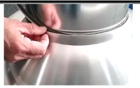
Back on the roof, install **weather dust gasket** between **flashing** lip & reflective **tube**. Gasket gives tube room to rise and fall slightly as it heats up, also preventing bugs and debris from getting inside.
