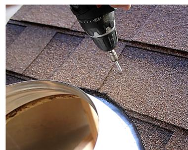
Completely coat screw heads and exposed edges between flashing & shingles with roof sealant.
