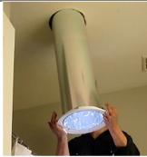
Slowly fasten **ceiling ring screw tabs**. **Ceiling ring** has self-tightening wing nuts to connect with drywall. *Do not overtighten*.
