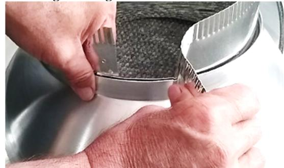
Install **dome assembly** over **flashing lip** and fasten with **#8 x 1/4" dome screws**.
