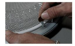
Take connected **tube** sections and fasten with crimp edge down over tube starter. *Make sure crimp edge is completely covered by tube starter*. Connect using (2) **tube screws and aluminum foil tape**.
