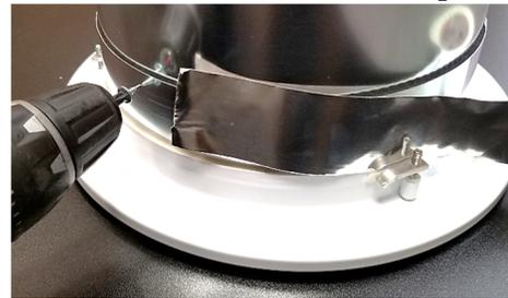
*Optional: You can also fasten just (1) **tube** section to **tube starter/ceiling ring** and install remaining **tube** sections from the roof. Then fasten sections from inside attic with (2) **tube screws & aluminum foil tape**.*
