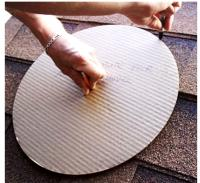
Using a **reciprocating saw**, cut along the traced circle through the roof material, tar paper & wood panel.
