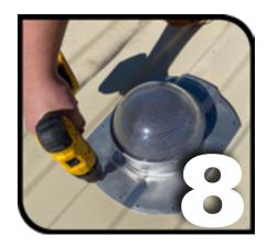
Step 8: Attach LightBlaster with Screws
