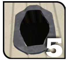
Step 5: Attach the Foam Gasket
