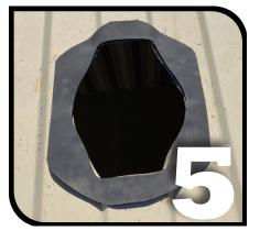
**Step 5: Attach the Foam Gasket**
