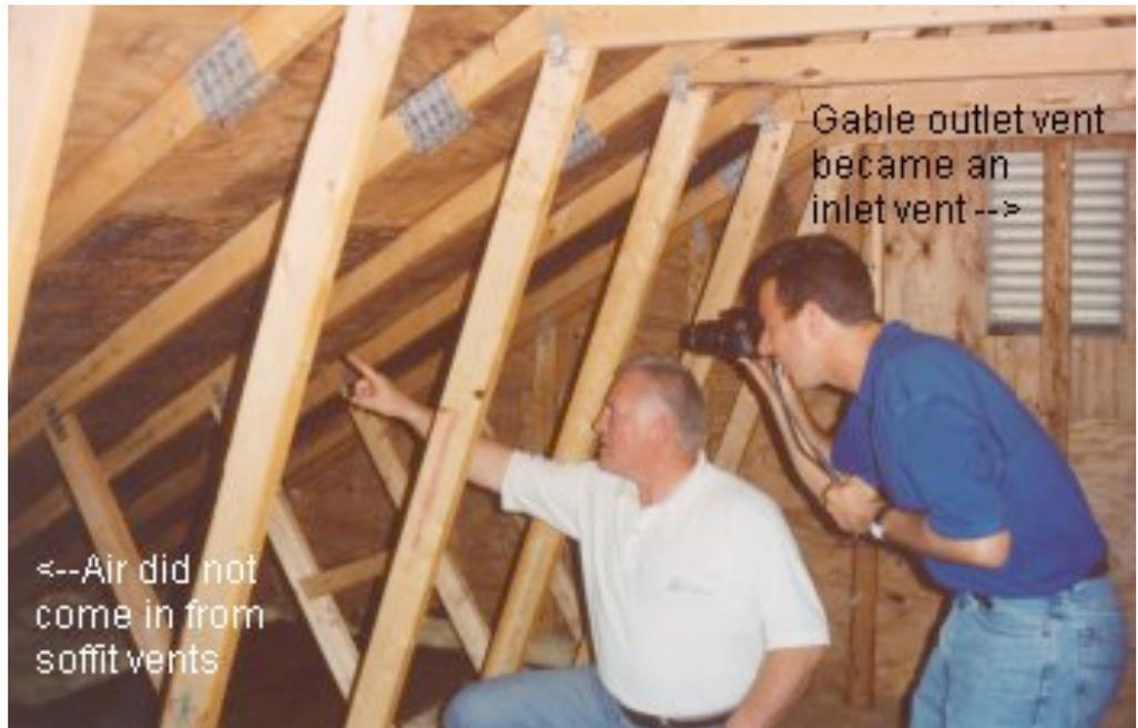
flowing, along the entire underside of the roof's sheathing, gathering up and removing water vapor.
